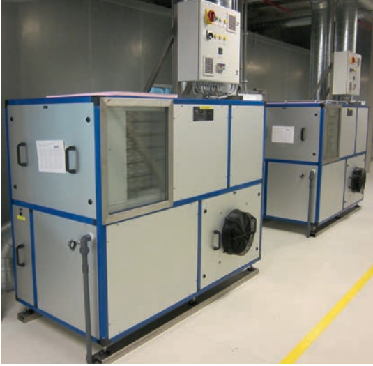
Two compact condensation drying systems provide adequate air-conditioning for the painting process. Dry air is passed over the items to be dried absorbing humidity in the process.
