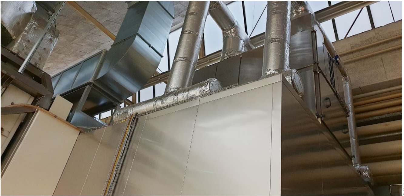
The dehumidification module is placed above the drying chamber for space restrictions.
