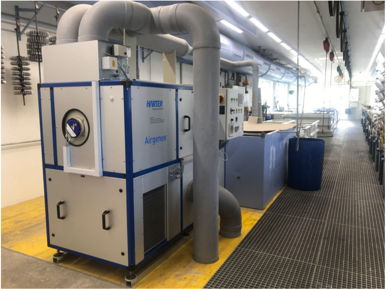
The dehumidification module conditions the process air required. The inbuilt heat pump technology is energy-efficient enough to qualify for government subsidies.
