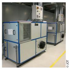
Two heat pump modules condition the process air to provide the correct environmental conditions for the drying process. Extremely dry air is passed over the items to be dried to remove humidity – at low temperatures.
